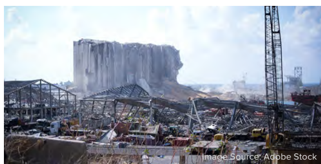
Photo 2: Destroyed buildings from Beirut's port explosion
